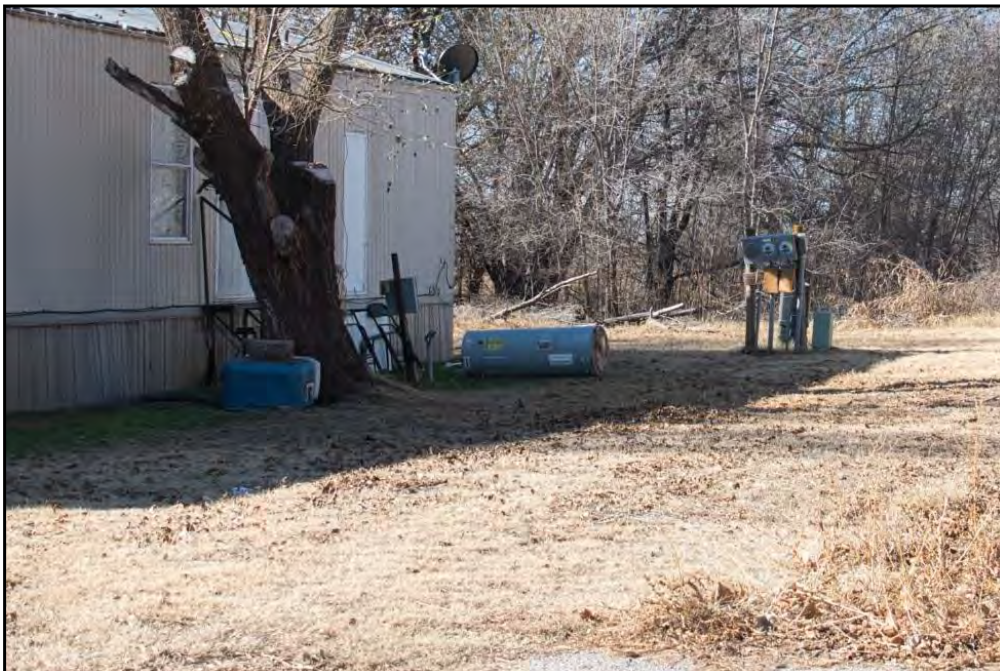
Water heater beside vacant mobile home on west side of S. Elk Ave
